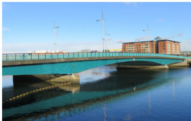
Gambar 2.4 Jembatan Gelagar Besi Queen Elizabeth II
